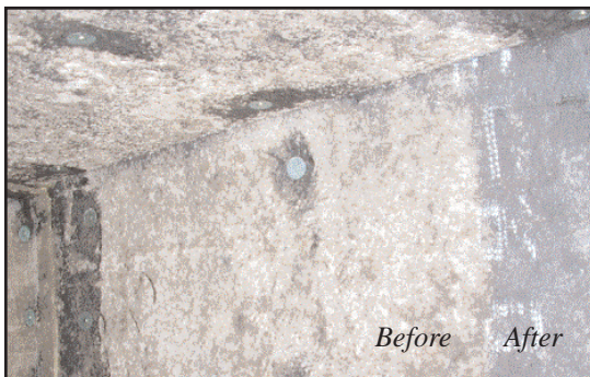
Ductwork before & after HEPA vacuum treatment
