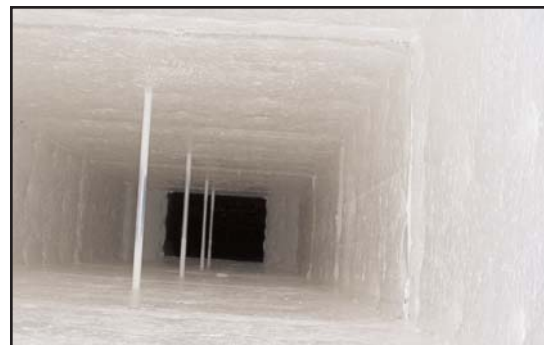
Ductwork after high performance repair coating
